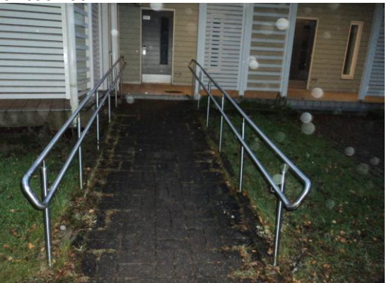
Ramp to ground rooms
